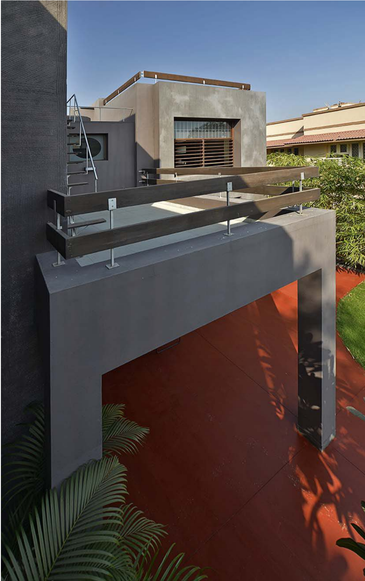
Roof of the verandah used to form a terrace space
